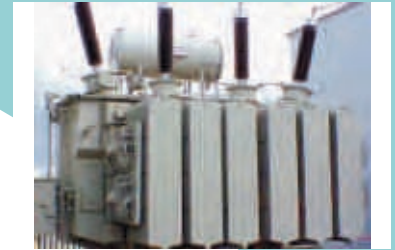
25 MVA, 110/11 kV NEW ZEALAND
