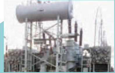
160 MVA, 220/132 kV MPPTCL
