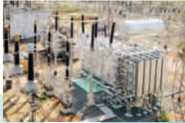
160 MVA, 230/110/11 kV TANTRANSCO
